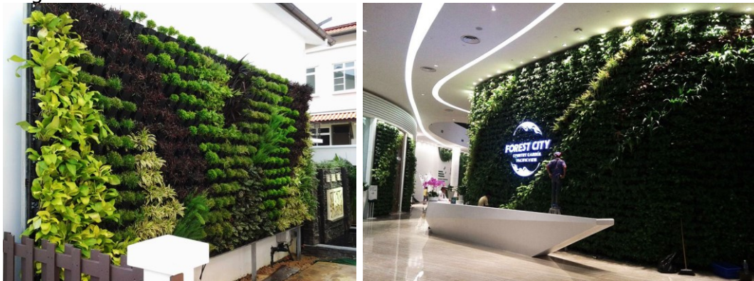
Figure 5: Example of modular living wall in Malaysia (Source: Hydro Solution)
