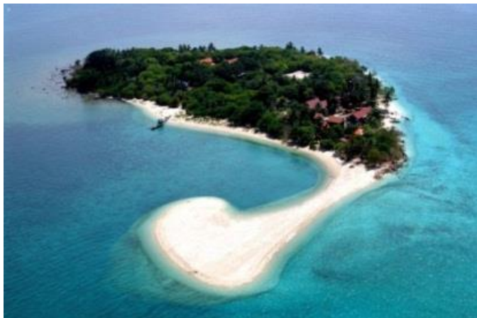
a. Formation of spilt at the southern part of Selingan Island before the shoreline protection.
