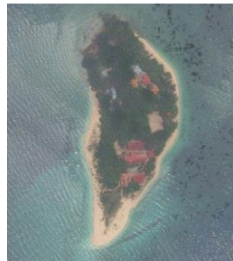
c. Spilt has disappeared and sand accumulated at southern end between the shoreline protection and the Island.
