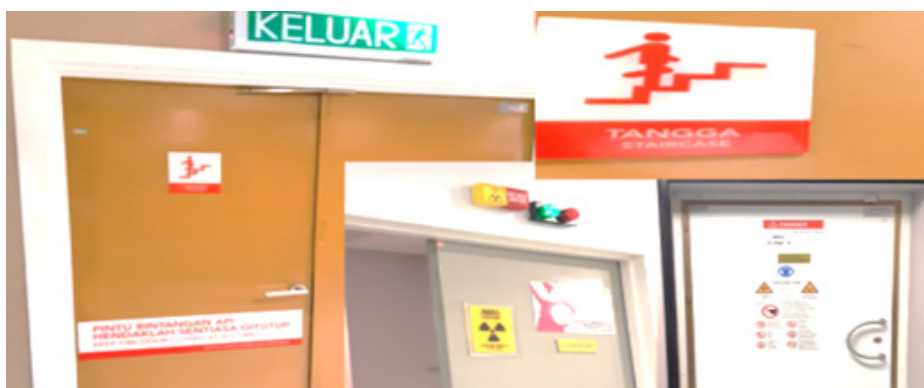
Figure 6 Gleneagles Kota Kinabalu Hospital warning signages
