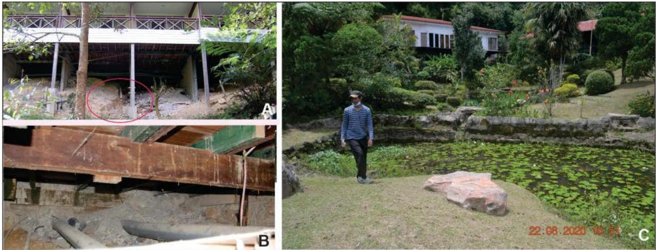
Photo 6 Subterranean erosion. A- water leakage (red circle) due to broken channel or connection failure: B- subterranean drain (PVC) that is connected to the river; C- a small pond that is connected by the subsurface concrete drain. This pond is believed to be a small old river channel that fills and alters into a subterranean concrete ditch.
