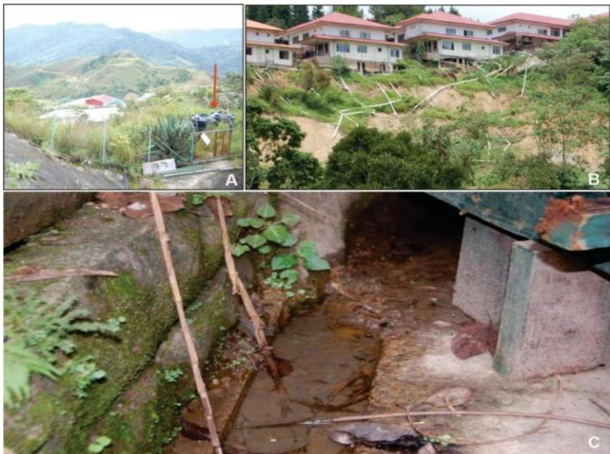
Photo 7 Water leakage from utilities. A- water tank to reserve water supply; B- part of irrigation or drainage system around this Resort; C- concrete ditch filled with water shows a fault (?) form fracture.
