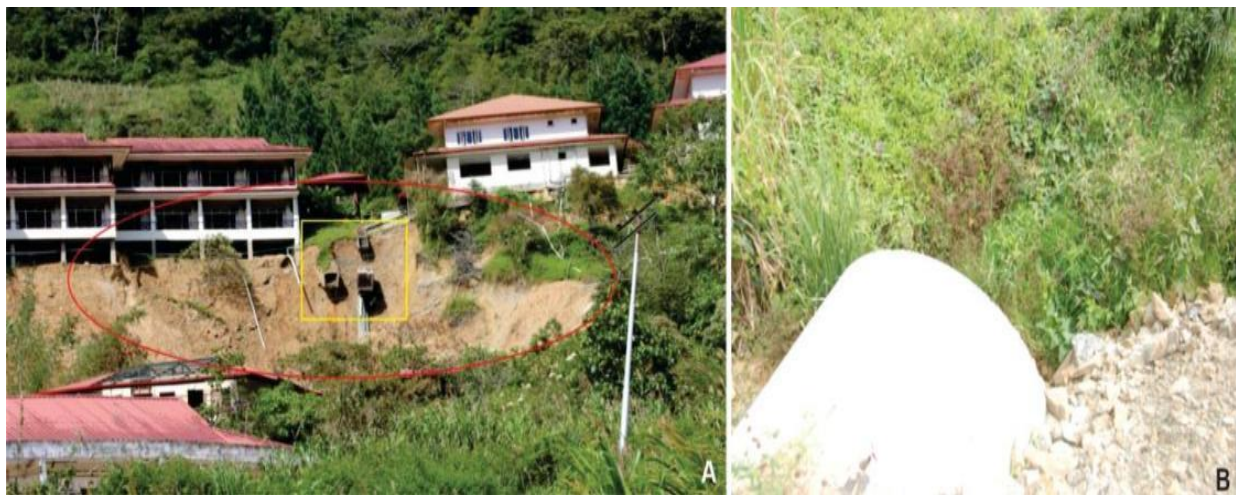
Photo 5 A- Evidence of old drainage channel and landslide which has been cut (for foundation and building) and filled (red circle) and alteration of natural drainage by the construction of concrete drainage (yellow square). B- filling activity and changing natural drainage channel into the culvert.
