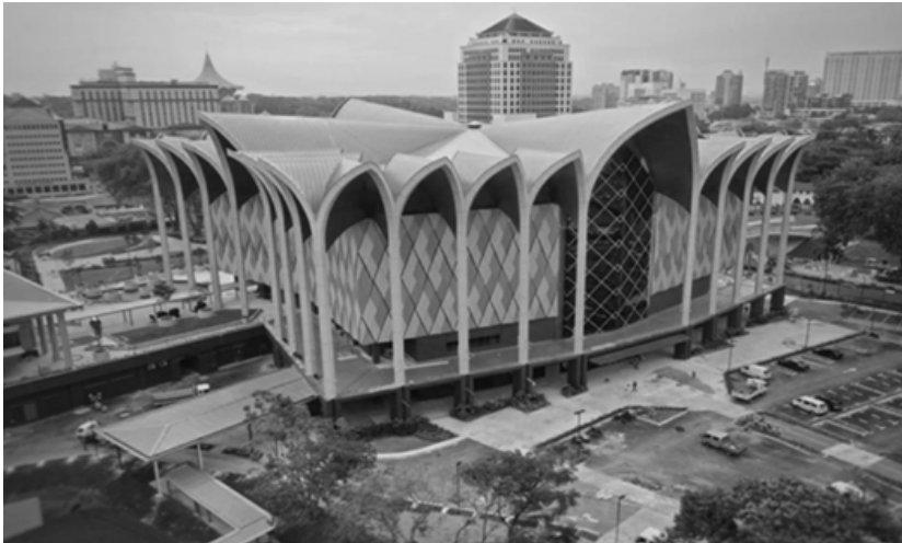
Photo 2 The New Sarawak Museum Complex
