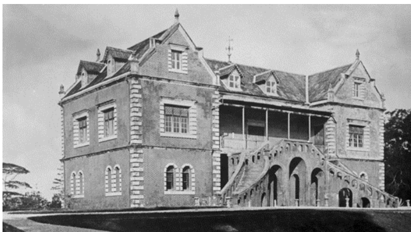
Photo 1 Museum Sarawak, old building
