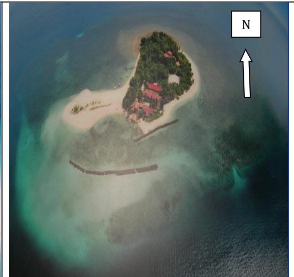
Figure 2c: Aerial photo of Selingaan Island in 2008 (Sabah Parks, 2011). Reef ball and stone revetment are built at the south of the island. Arrow indicating North.
